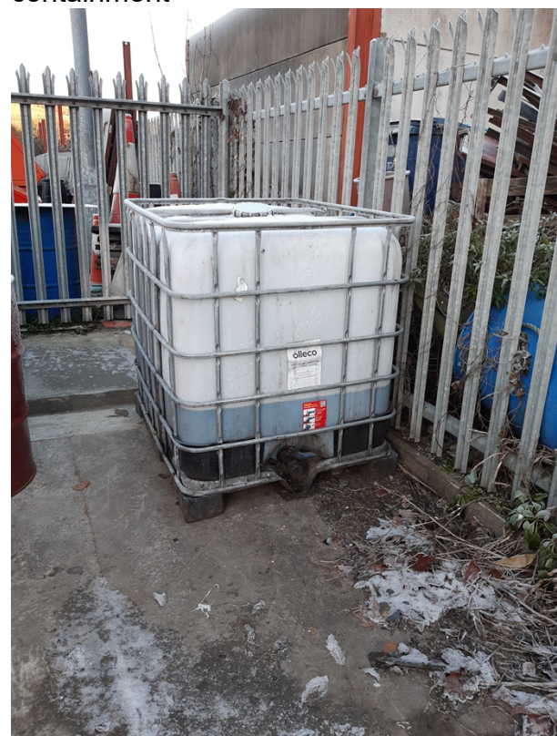
Cooking oil - which was being kept on site in a single skinned container without secondary containment
