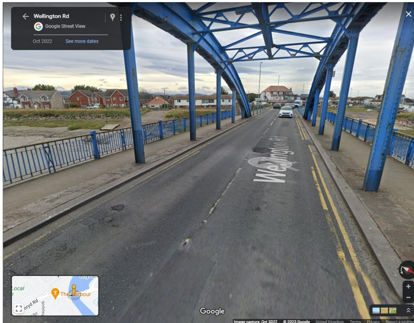
2. Western extent of bridge deck. (Source: Google)
