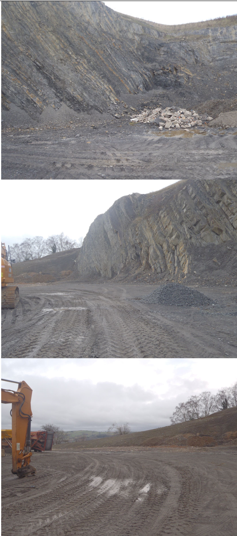
Photos showing deposits of aggregate on mostly clear site
