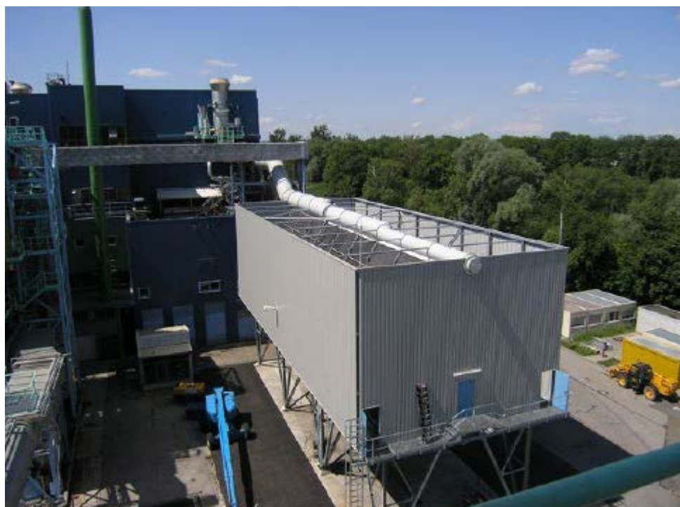
Figure 3.2 Air Cooled Condenser
