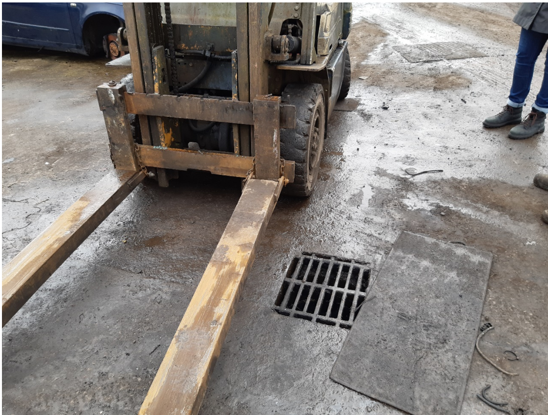
Photo 2 – drain cover within operational area of yard.
