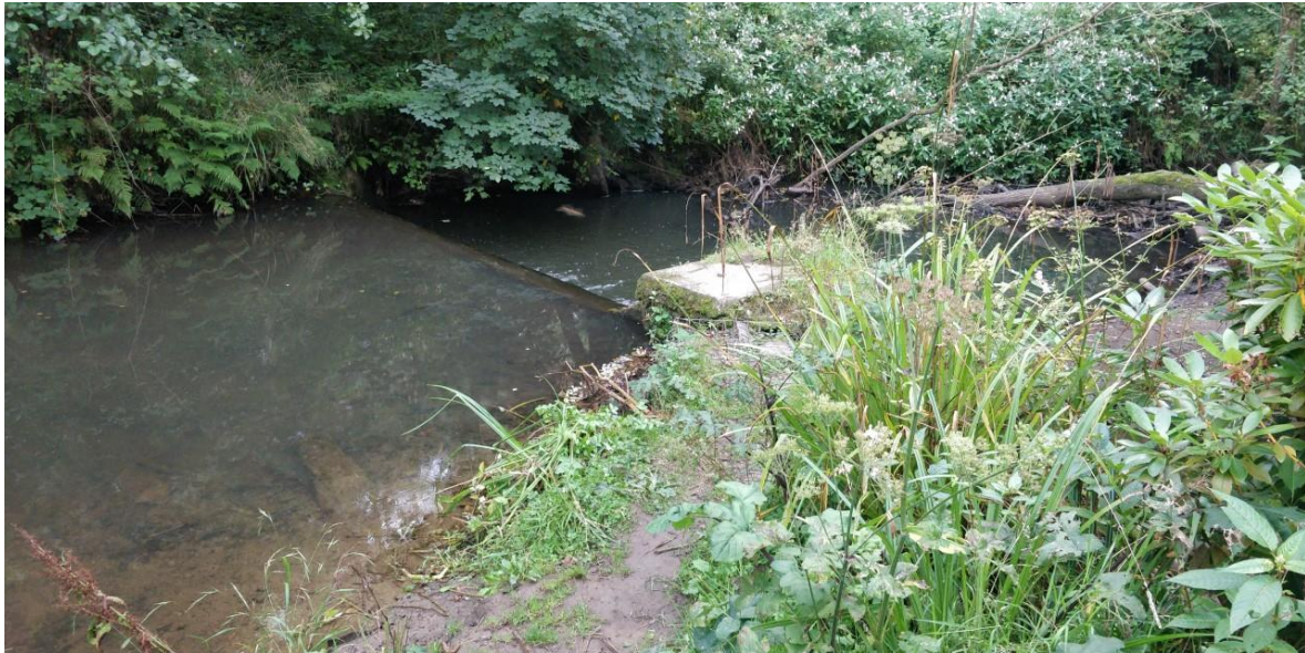
Figure 3. The most upstream weir to be removed.
