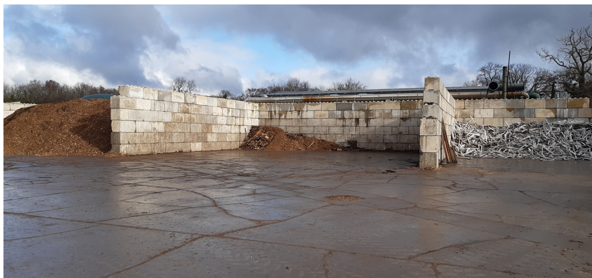
Photo 5 - Stockpiles of wood and uPVC waste(s) stored within segregated concrete bays
