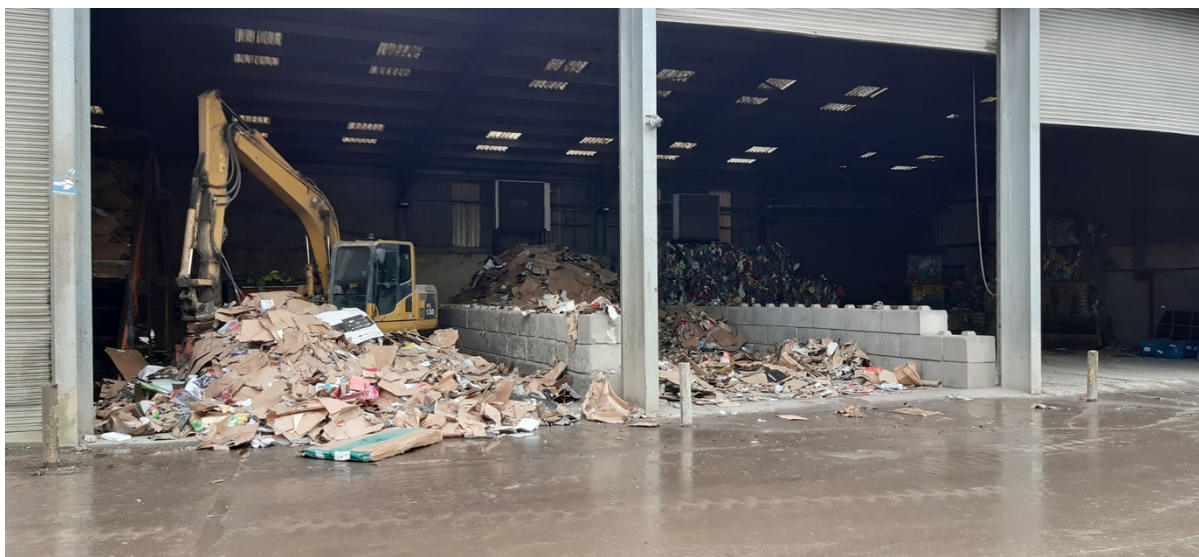
Photo 3 - View inside waste transfer station building
