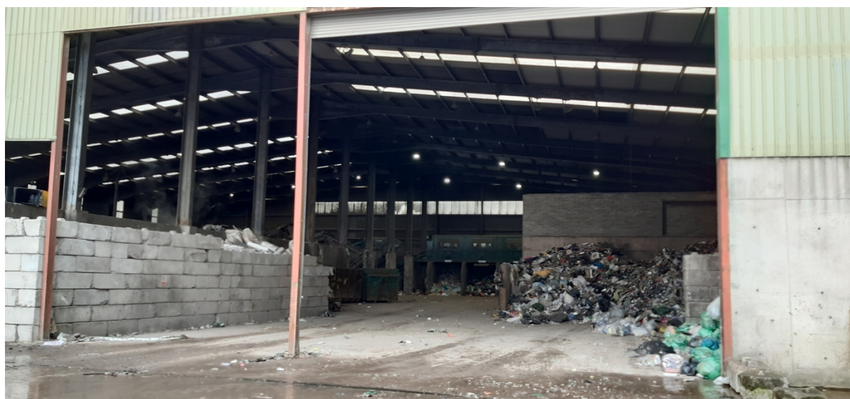
Photo 1 - View inside waste transfer station building
