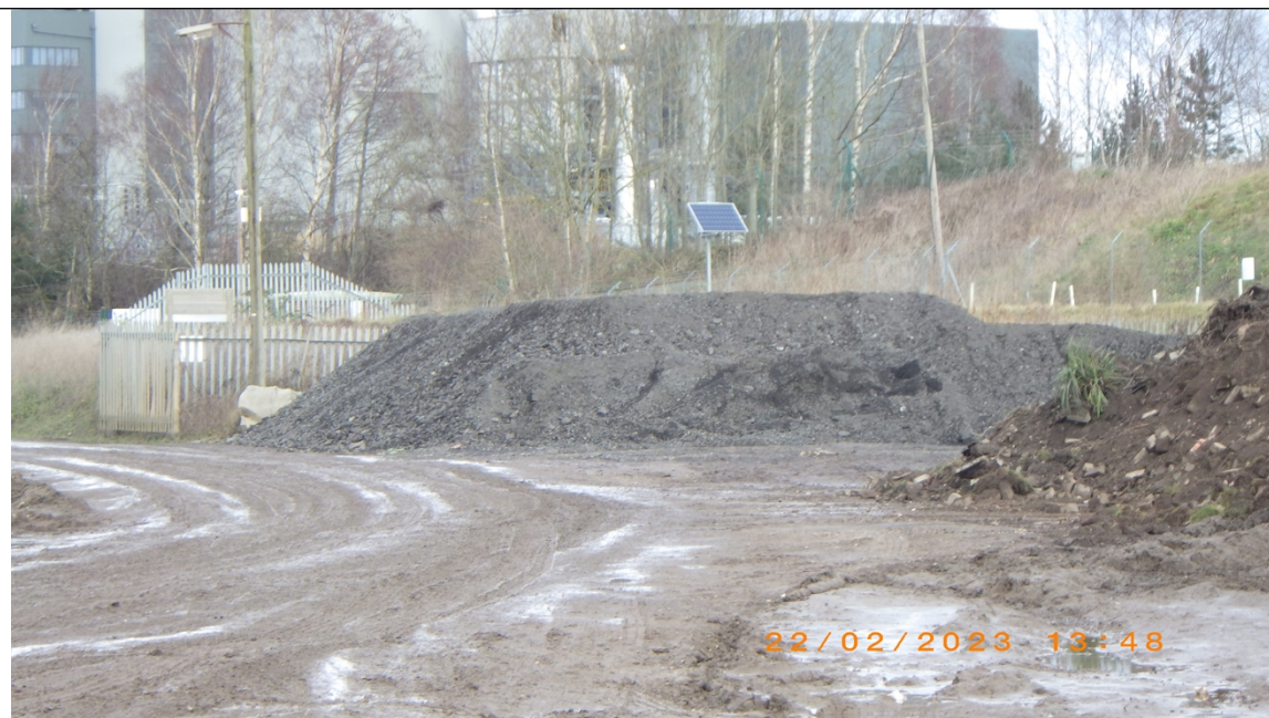
Photograph showing storage of road planings
