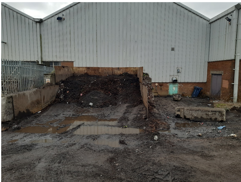
Photo 2 – to the right of the dewatering bay shows escape of water away from drainage channels.
