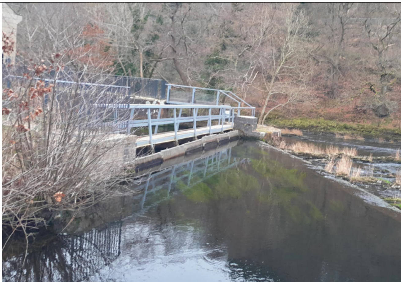
Air blowers operating to prevent screens from blocking
