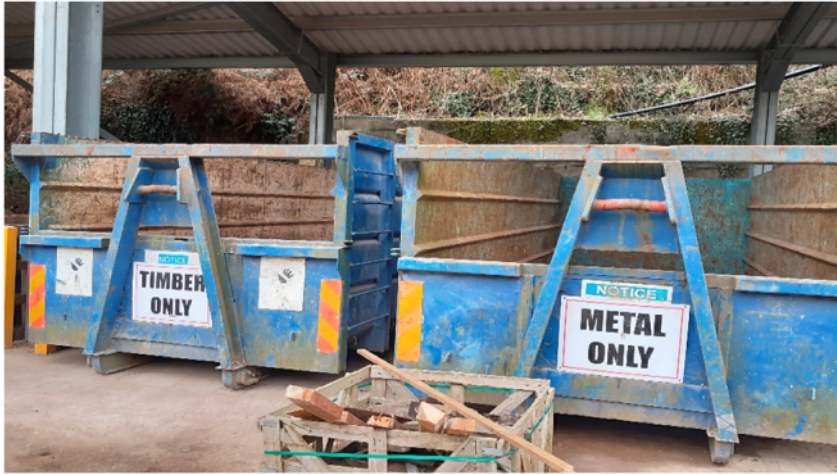
Image 1 & 2 showing separated skips with the different waste streams stored within the building recently constructed.
