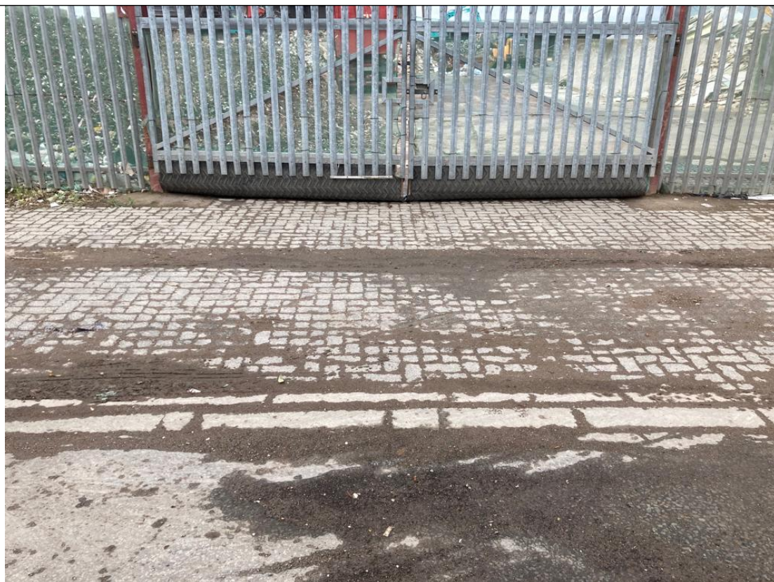
Photo 2 - Newly installed excluder on access gate at GD Environmental, Newport
