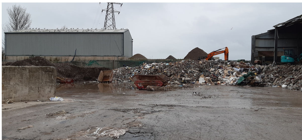
Photo 4 - Weakened areas of concrete flooring at GD Environmental
