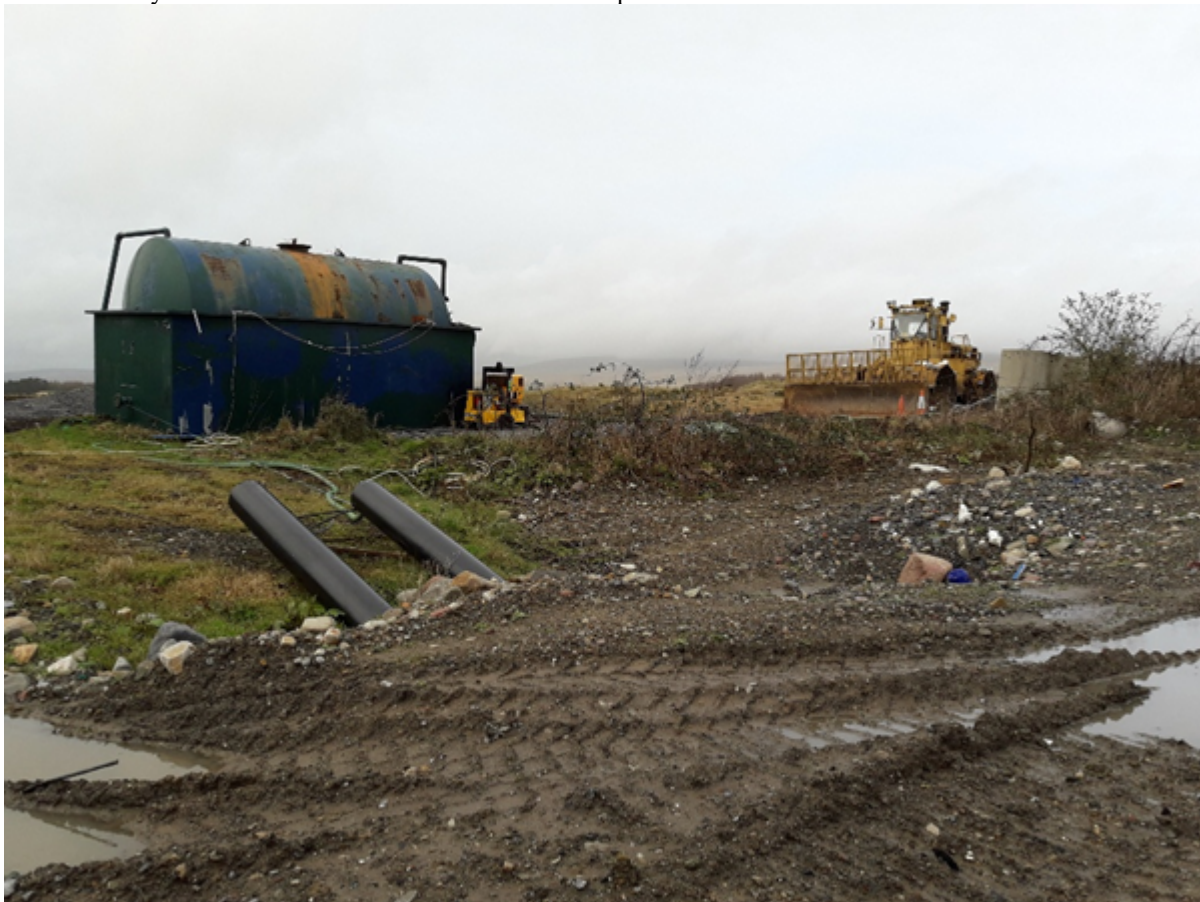
Photo 4 showing Valley Infill and leachate infrastructure.
