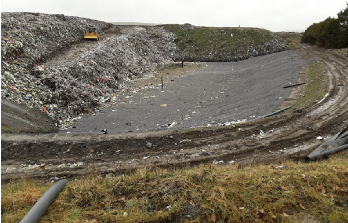
Photo 2 showing sub cell 6 and waste encroachment
