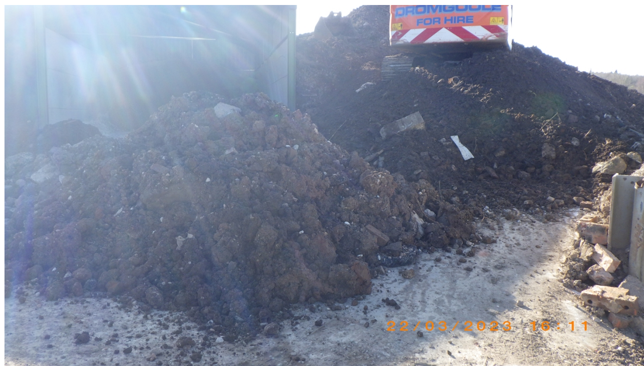
Photograph showing inert waste storage
