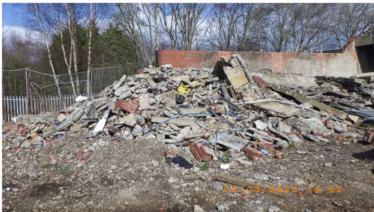
Photo showing demolition waste formed on site
