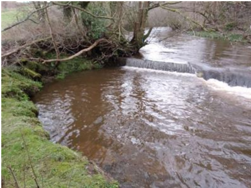
Figure 14. SN 62163 10669 Erosion DS of weir. Taken facing US from RHB.
