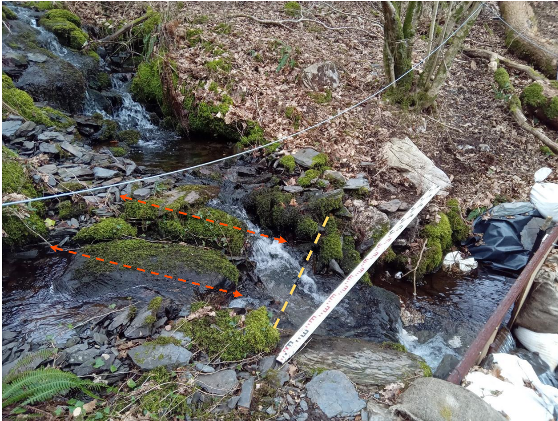
Weir located at natural fall in watercourse in order to create limited impoundment volume (shown with orange arrows)
