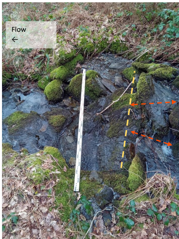
Weir located at natural fall in watercourse in order to create limited impoundment volume (shown with orange arrows)
