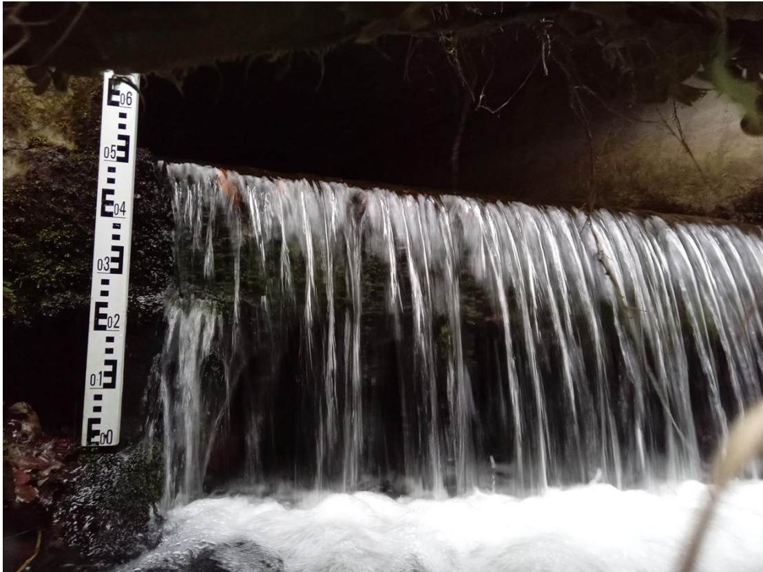
33. Grid Reference: SH 58506 41885 Outfall from culvert - 0.65m drop
