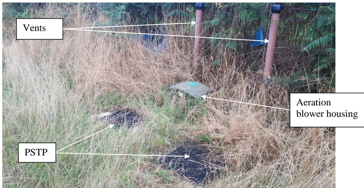
The secondary treated effluent resulting from this PSTP is pumped to a private drainage field. It is not possible to measure the size of the existing drainage field, but we can confirm that there was no evidence of pollution or failure at the time of our visit.
