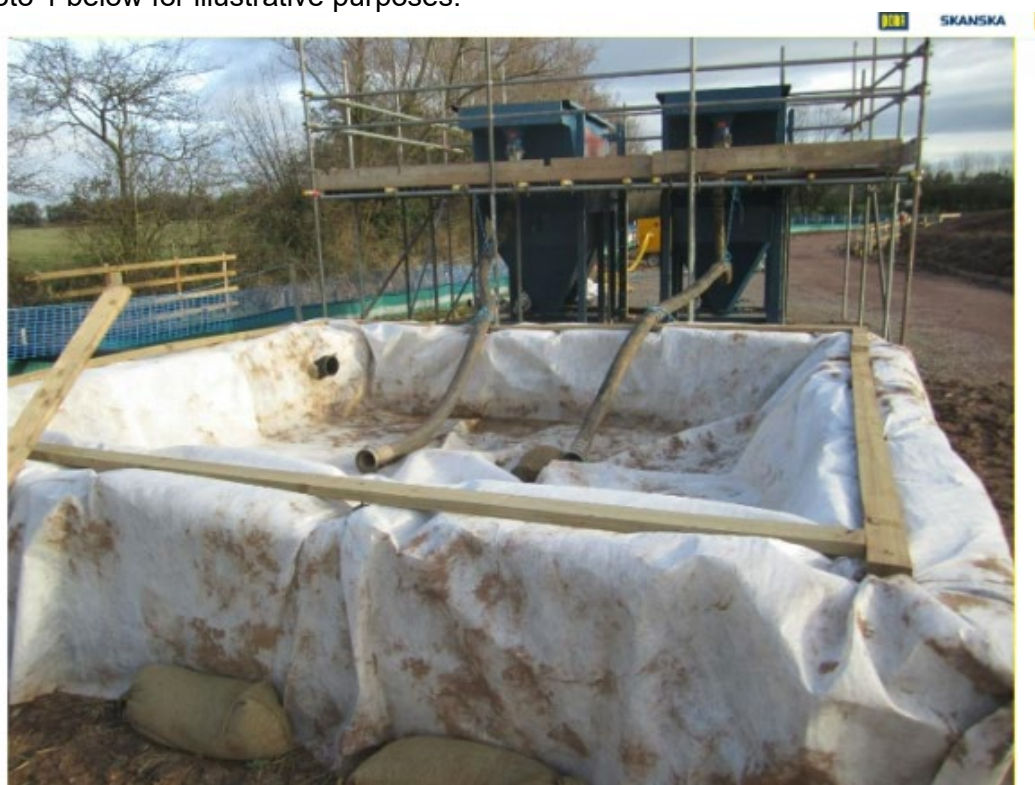
Photo 1 – Typical Silt Trap constructed of straw bales and geotextile membrane.
