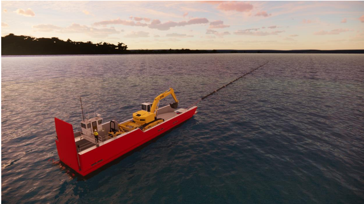
New pipe being transported from the harbour facility into the required position.
