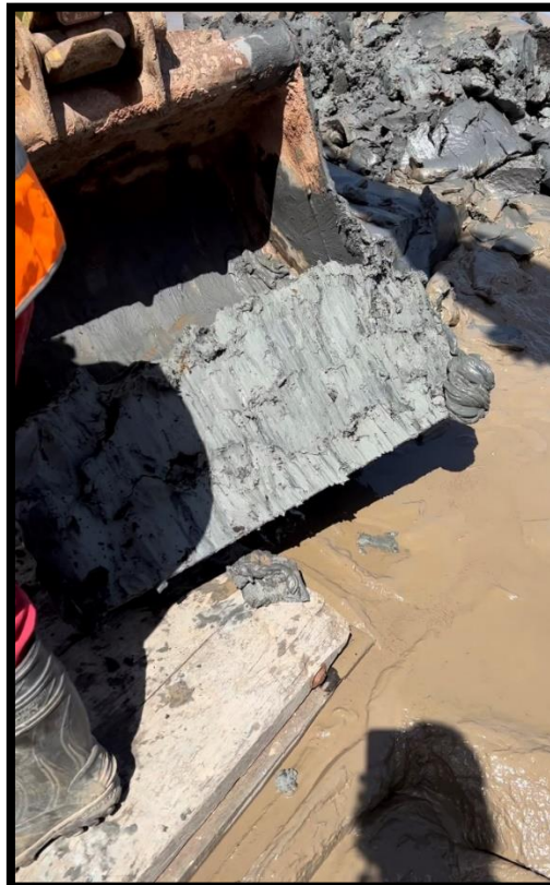
Photograph 9 – Taken during the Ground Investigation works- note the consistency of the underlying clay.
