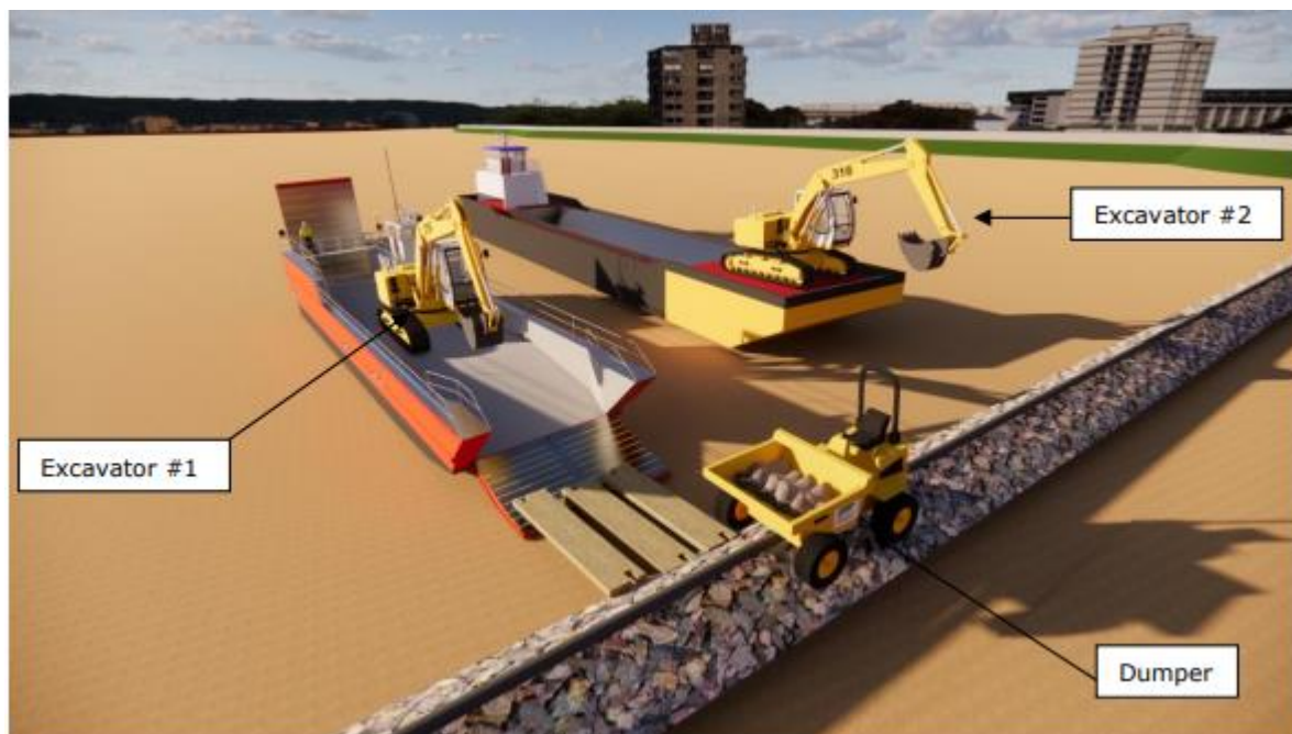
Figure 4 Illustration of working configuration during decommissioning of the existing pipe (reproduced from Kaymac 2022b).
