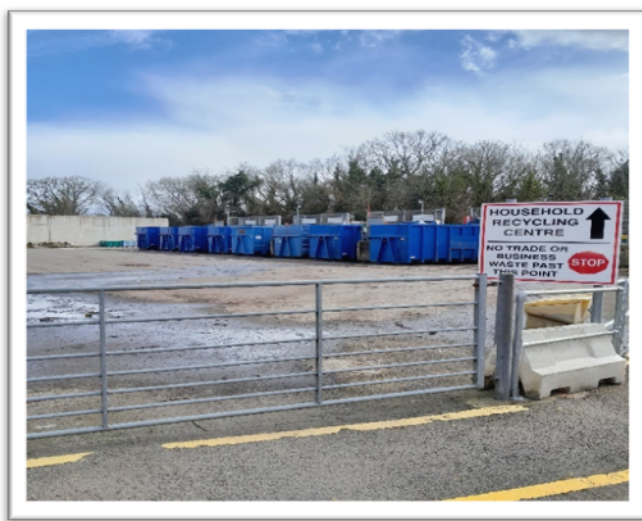
Photo 1 - Site flooring infrastructure in good working order with no concerns over integrity
