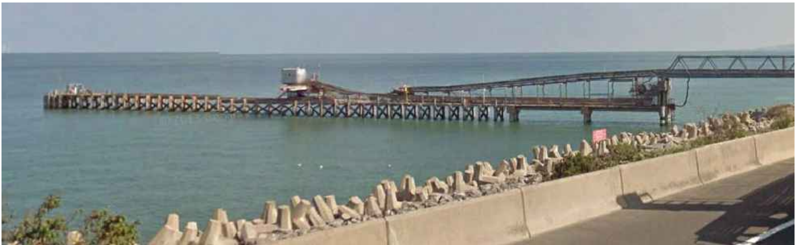
WEST SIDE GENERAL VIEW
