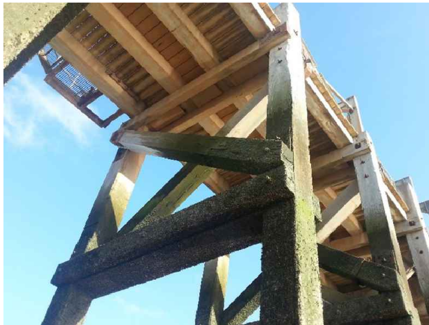
TYPICAL BAY VIEW FROM BENEATH
