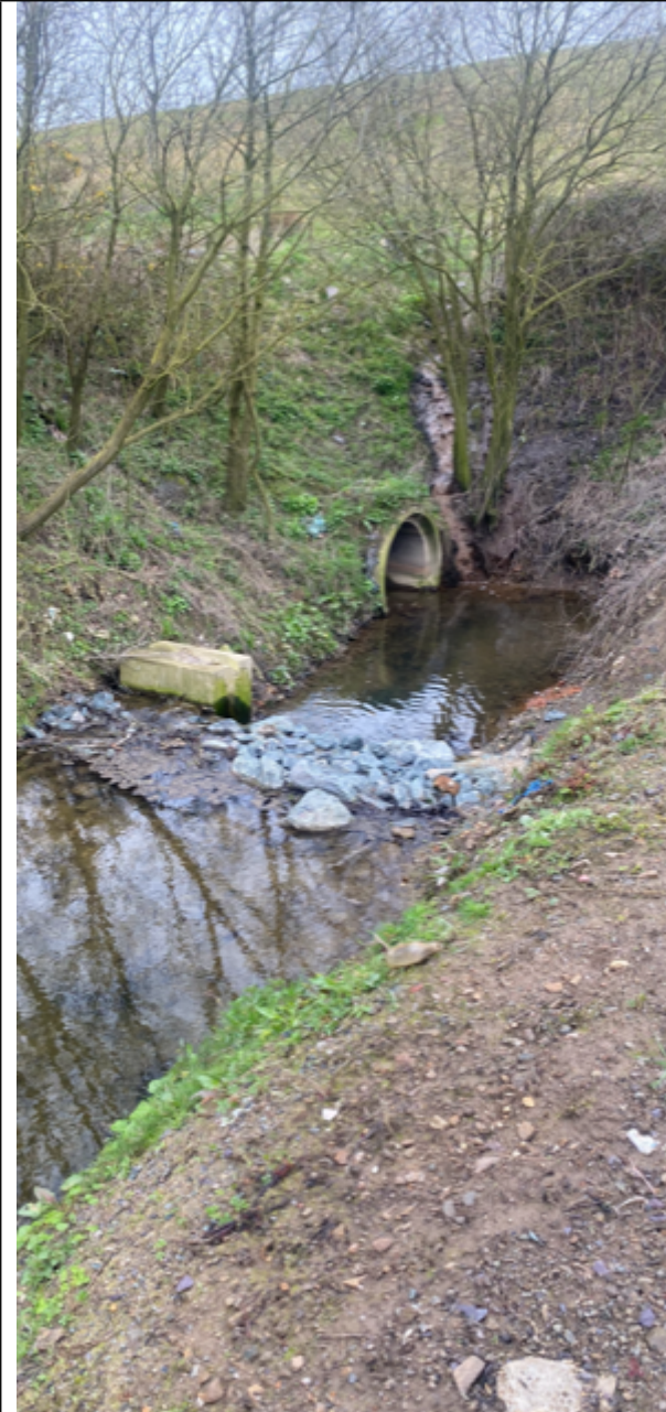
Photo 2. Penhesgyn Culvert Upstream and Silt Trap
