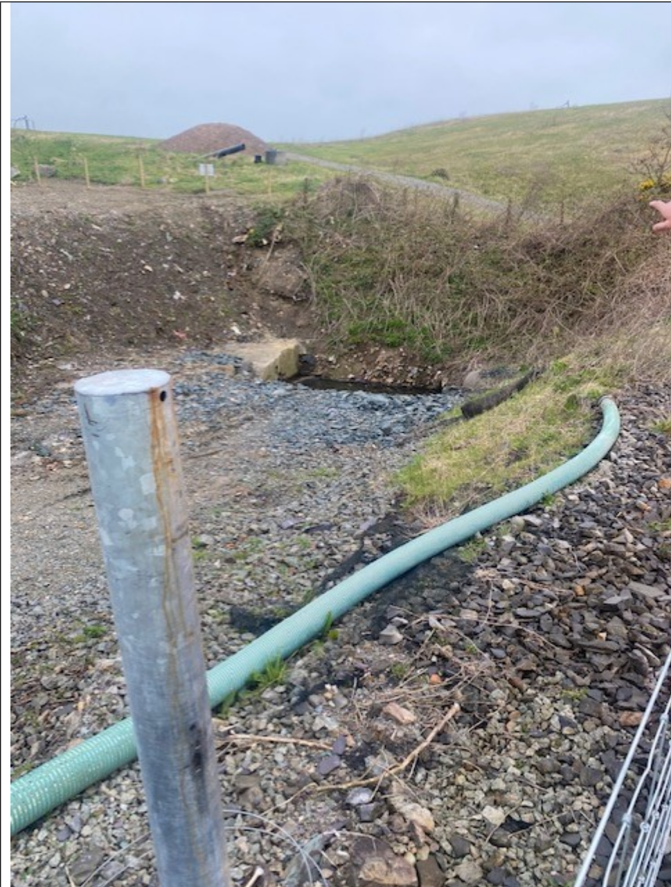
Photo 1: Penhesgyn Culvert Entrance.
