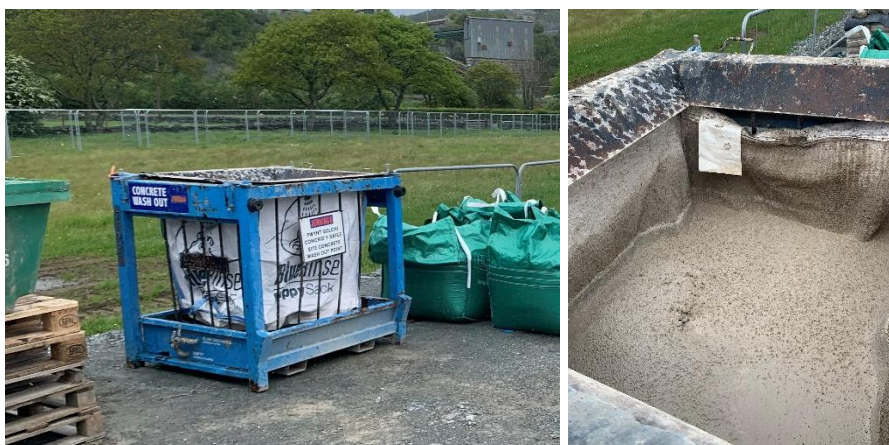
Figure B4 Concrete wash out skip at Garth site 10-05-23
