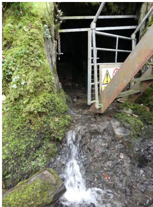
Figure 1 Existing mine water discharge from the Llechfraith Drainage Adit
