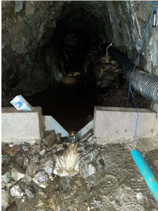
Figure 6 Second weir installed up-gradient of first weir. Note the black pipe on the right of picture carrying the diverted waters from the Upper Workings.
