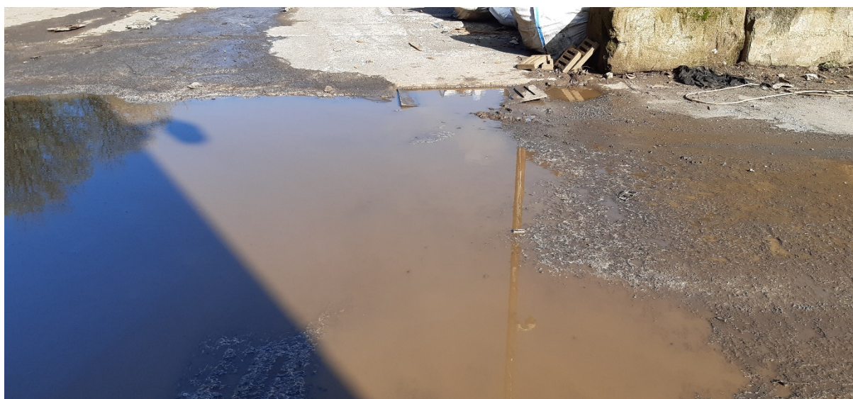
Photo 6 – pooling of surface water outside Unit 6
