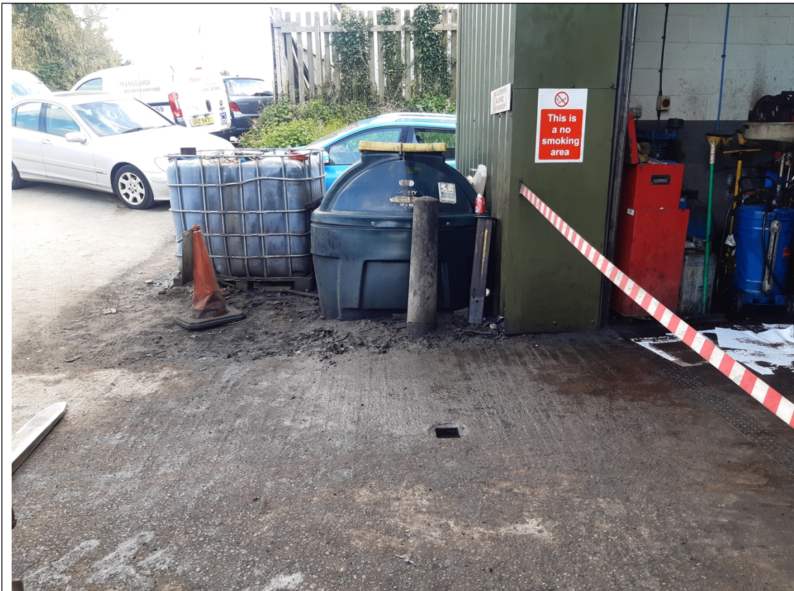
Photograph showing oils running from depollution shed onto unsurfaced ground
