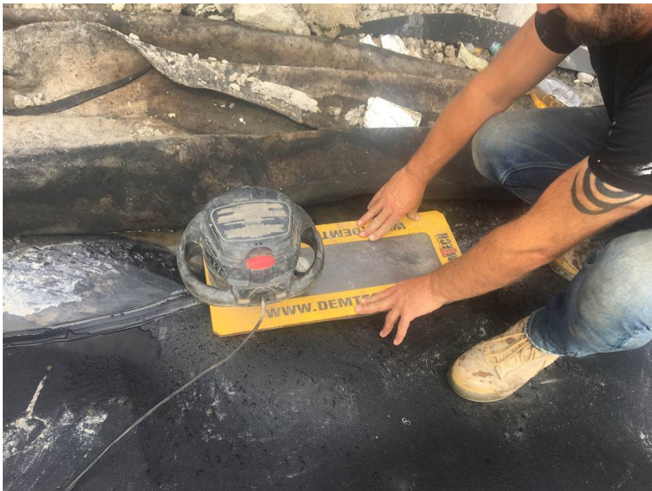
Vacuum box testing of HDPE
