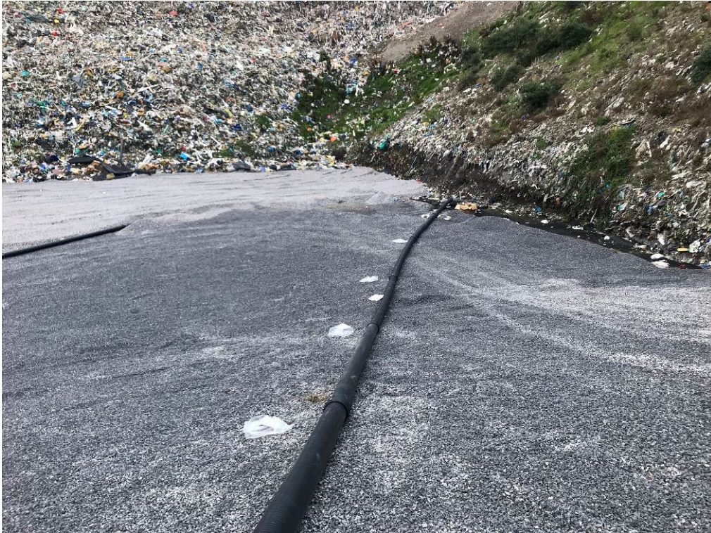
Spine drain extending from sub-cell 3
