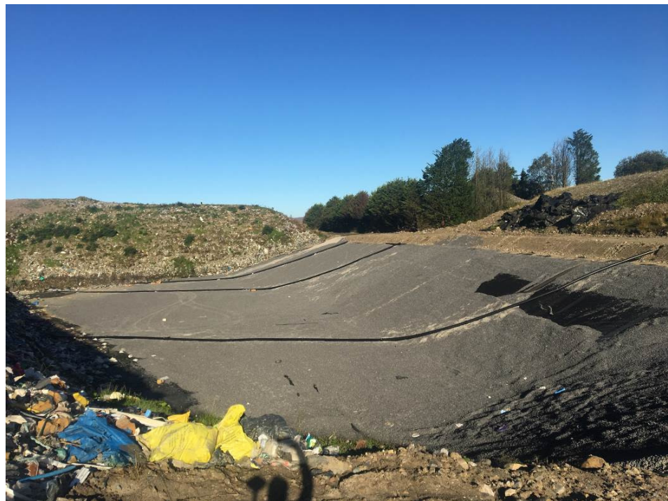
Drainage pipe runs on base
