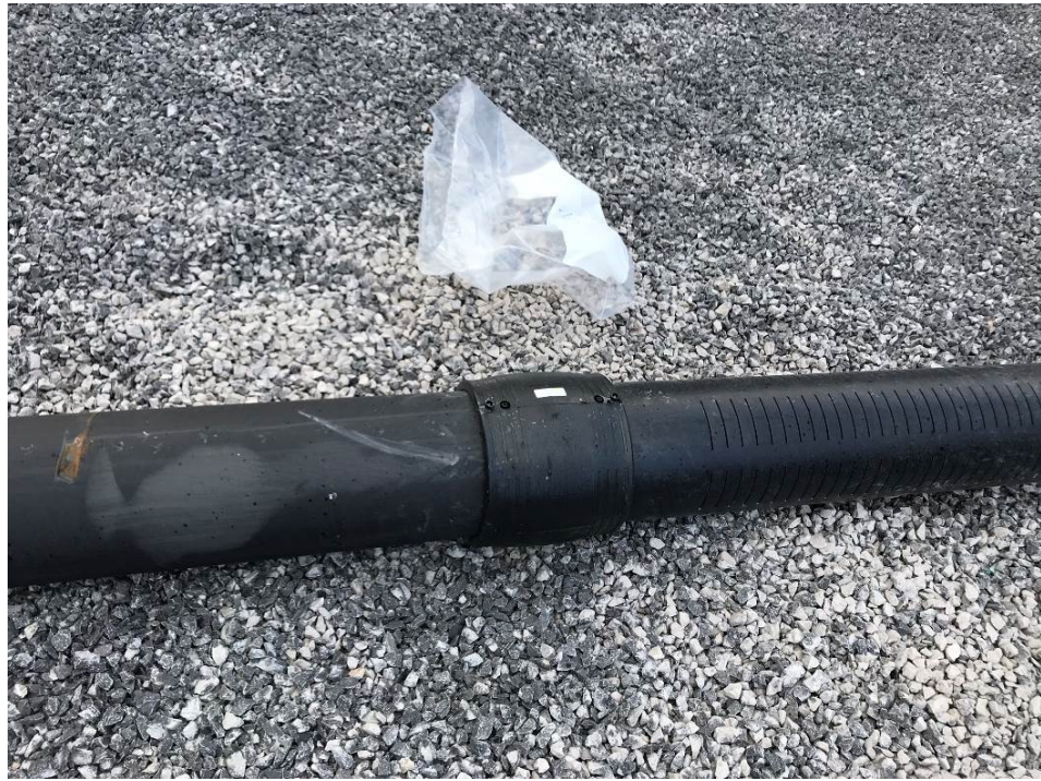
Drainage pipe with proprietary electrofusion collar
