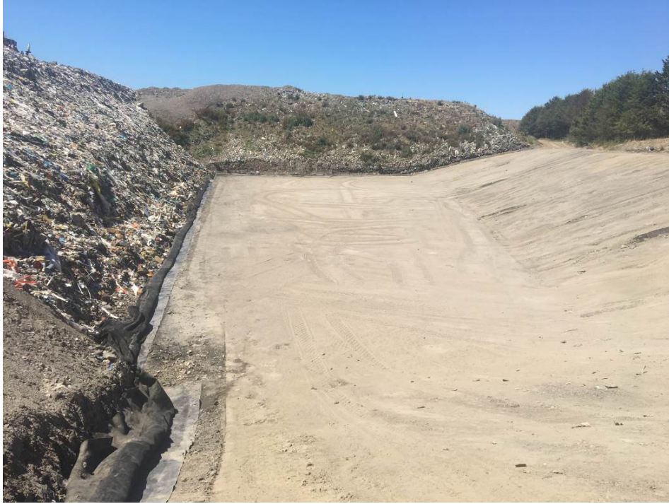
Mineral Liner on 29/06/18
