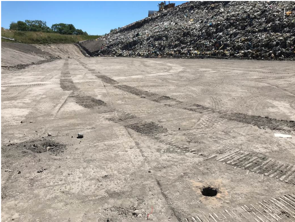
Mineral Liner with SRD test in foreground on 27/06/18
