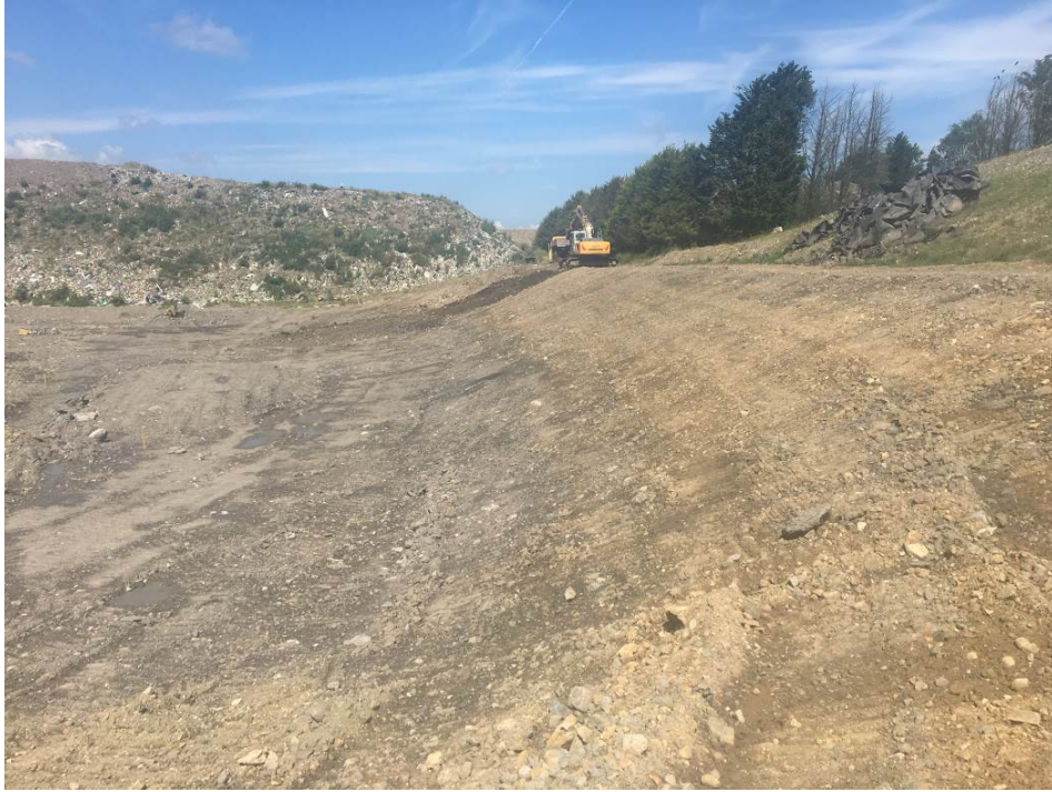
Formation construction on 11/06/18
