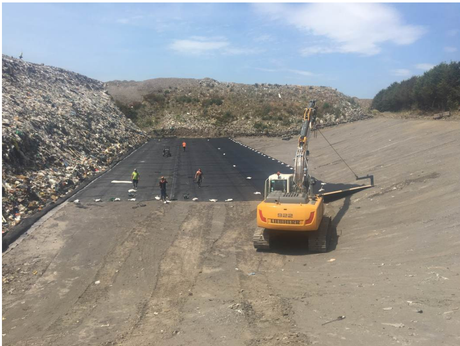
Commencement of HDPE placement on 2/7/18
