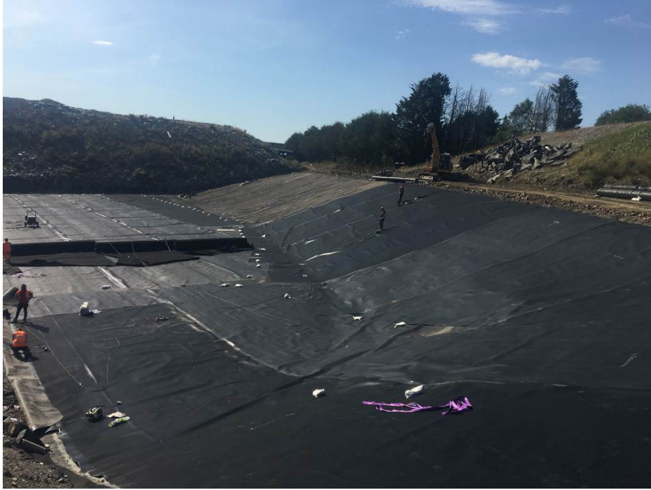
Deployment of Textured HDPE on side slopes
