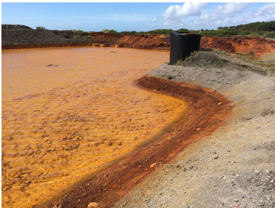
Plate 6-1 Cell 2 leachate sump L8. Note staining due to iron.
