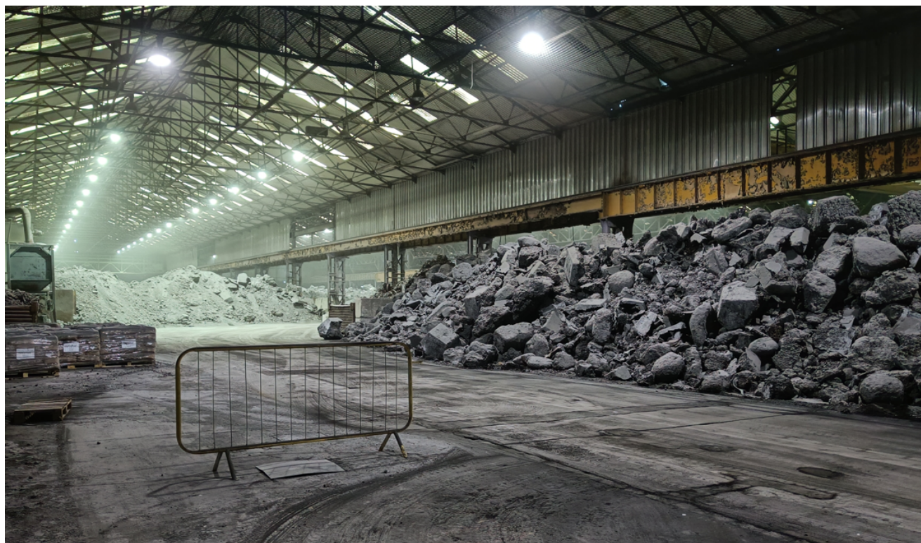
Salt slag storage area - lump slag in foreground, processed slag in background
