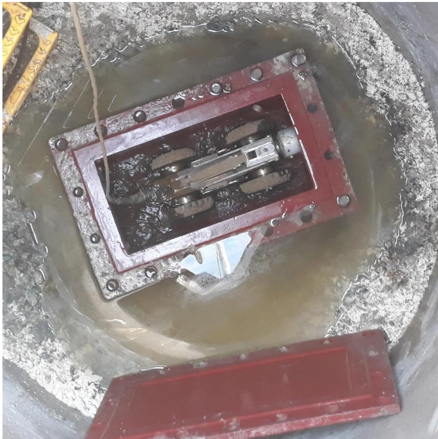
CCTV survey of pipe undertaken similar to previous survey shown here, from onshore chamber working offshore.
