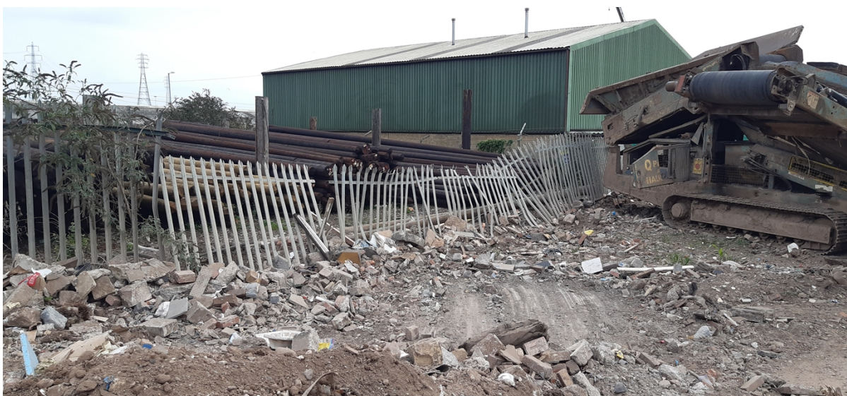
Photo 4 - Site fencing during site inspection on 01/09/22 (CAR_NRW0040365)
