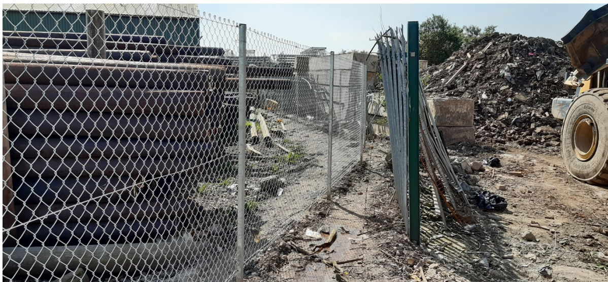
Photo 5 - Repaired security fencing at A1 Waste Management Ltd
