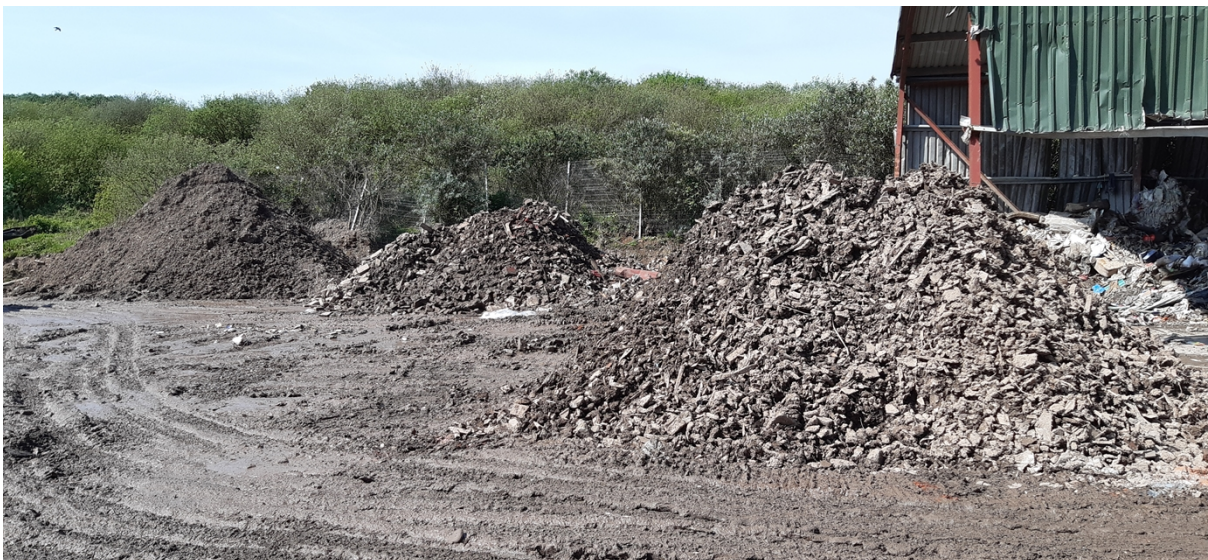
Photo 2 - Stockpiles of unprocessed waste in compliance with sites FPMP
