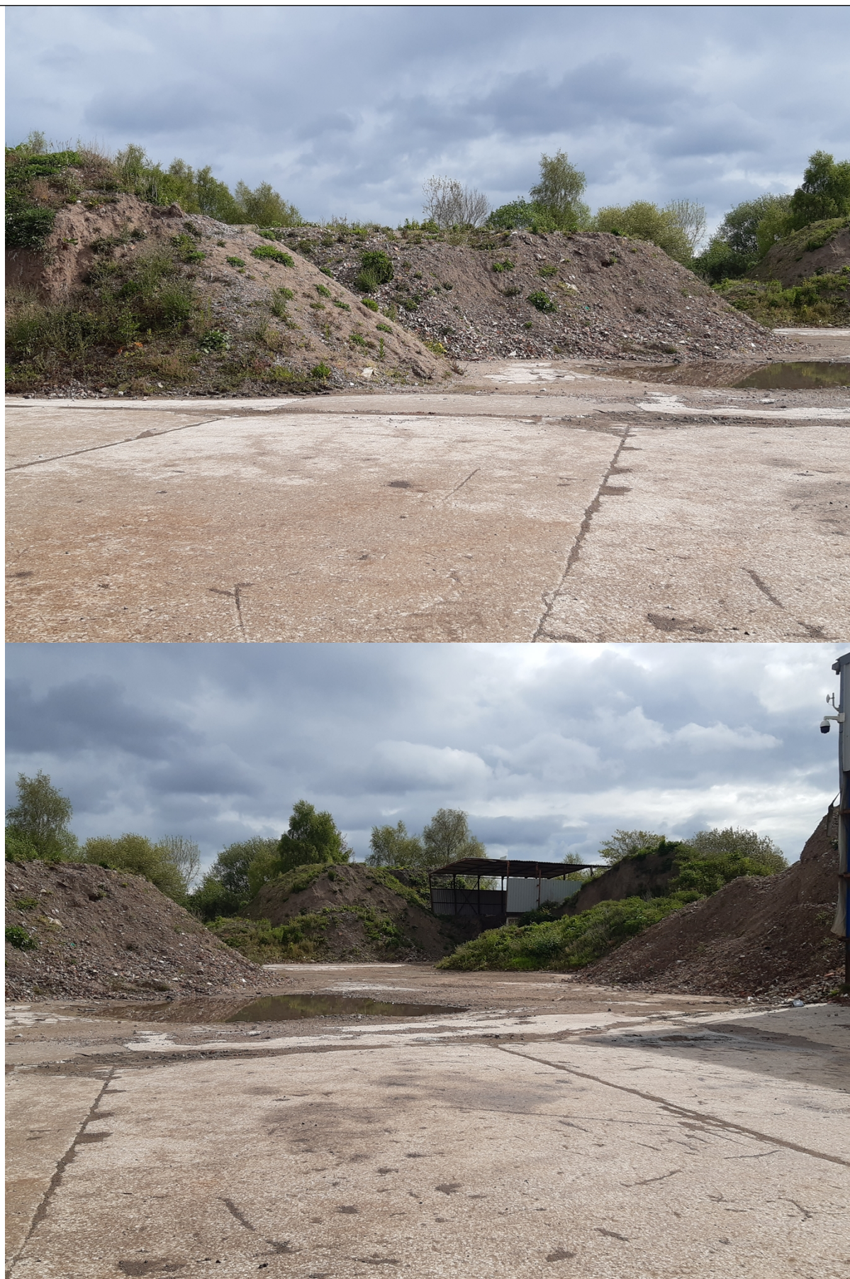
Photographs from site showing transfer building which remains free of waste and
