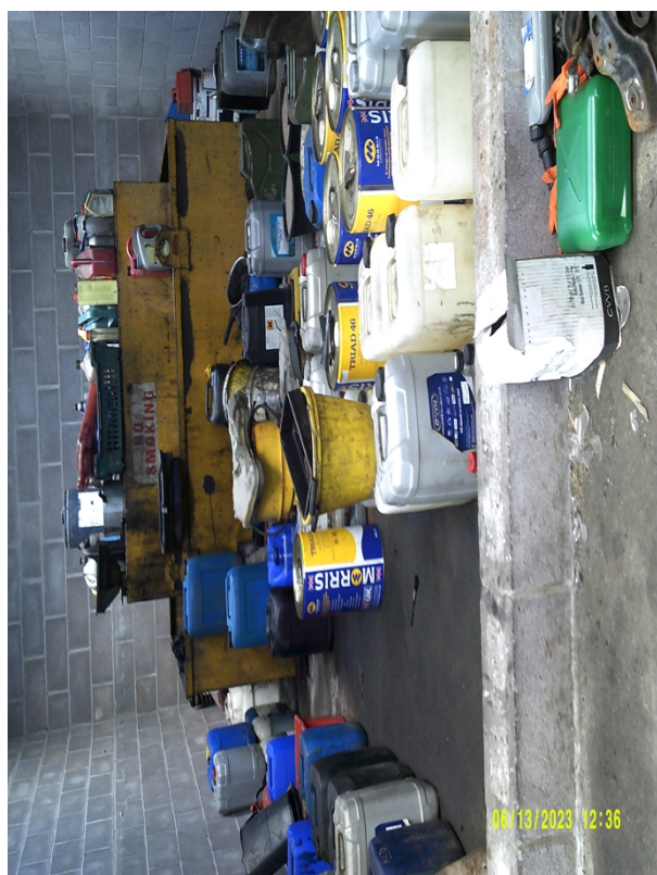
Figure 7: Bunded oil tank and other oil containers behind bund inside a building for storage.
