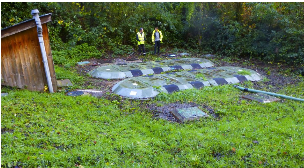
Photo of existing treatment plant installation showing two visible treatment tanks and 2 below ground tanks
