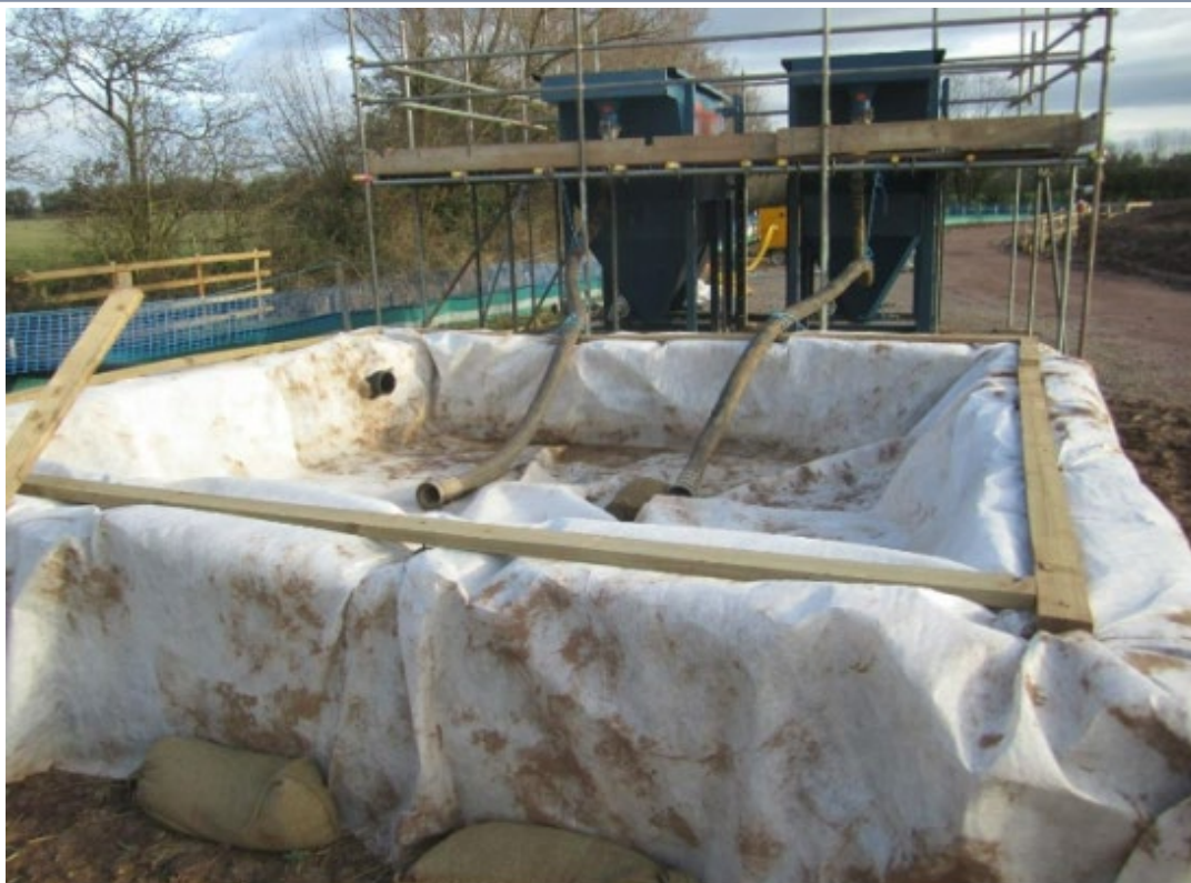
Fig. B6.4 Typical silt trap constructed of straw bales and geotextile membrane.
