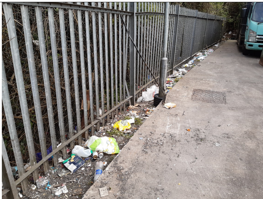
Photo 2 – the potential for litter to leave the site in busy areas of operation.
