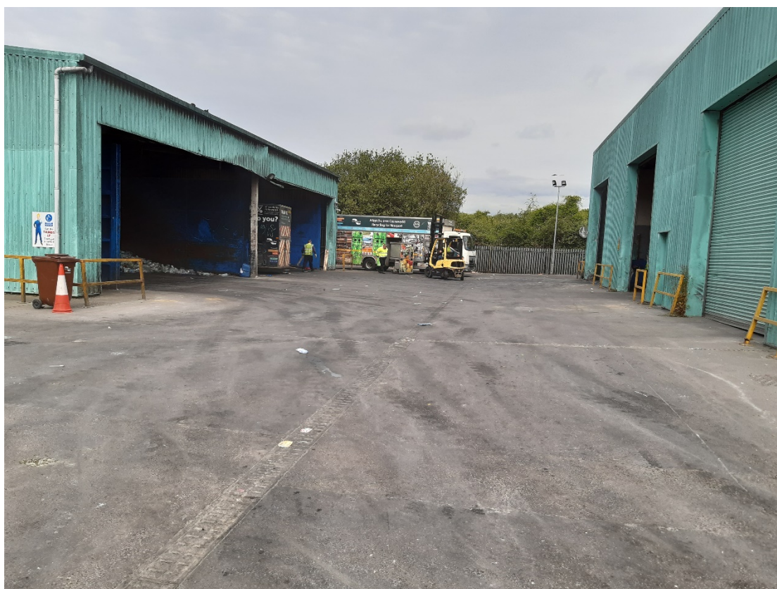
Photo 4 – yard area with no issues apparent with drainage/infrastructure on site at time of inspection.
