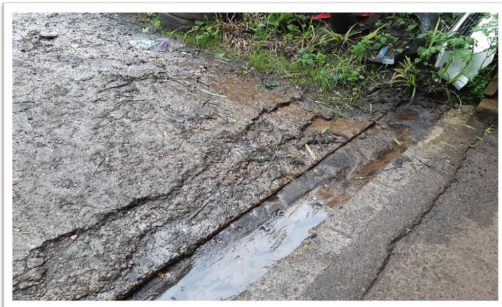
Photo 1 – Showing drainage channel with silt to be cleared
