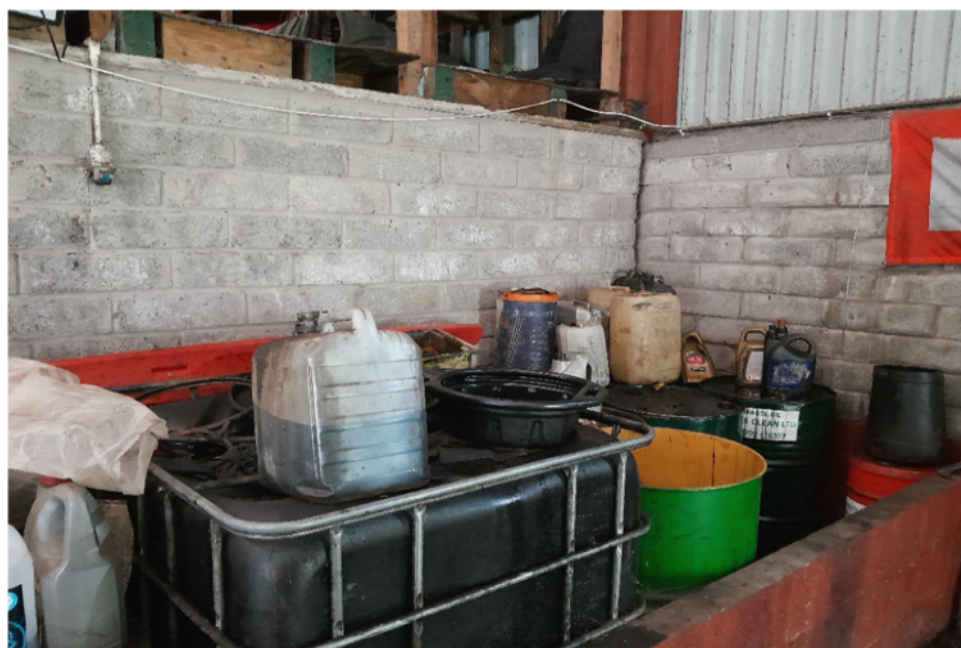
Photo 2 – Showing oil containers stored in the bunded area housed inside building
