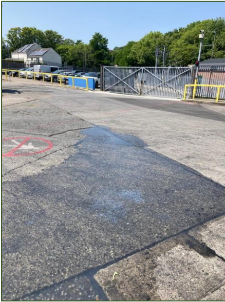
Photo 11 – proportion of flow towards the side gate drain.
