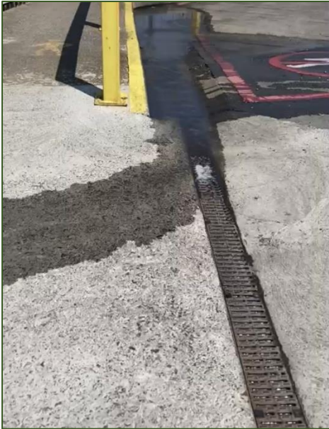
Photo 13 – proportion of flow towards the side gate drain. Small volume exceeded drain gully and flowed to gateway.
