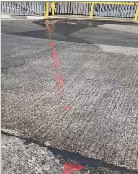
Photo 12 – proportion of flow towards the side gate drain.
