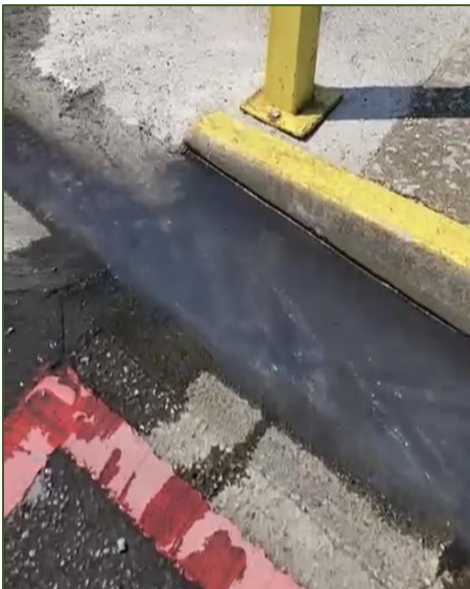
Photo 14 – proportion of flow towards the side gate drain. Small volume exceeded drain gully and flowed to gateway.
