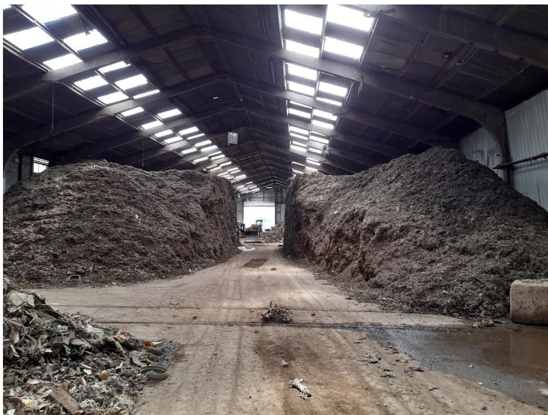
Photo 1 – access through the stockpile, see waste on left of photo is now 10m away from combustible material
