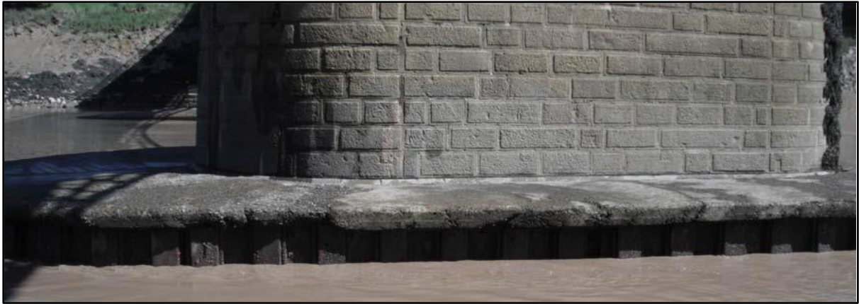
Figure 1.4 – Old Wye Bridge Pier 3, showing sheet pile base and concrete capping
