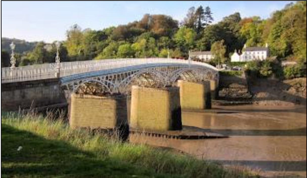
Figure 1.2 – Old Wye Bridge at Low Water
