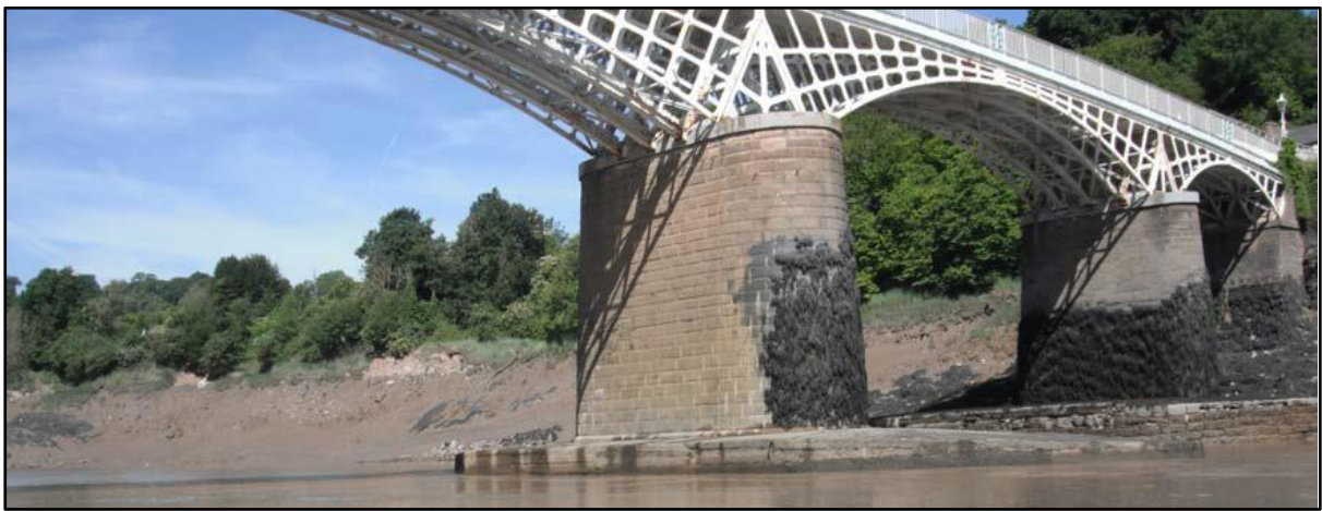
Figure 1.5 – Old Wye Bridge Pier 2, view from downstream
