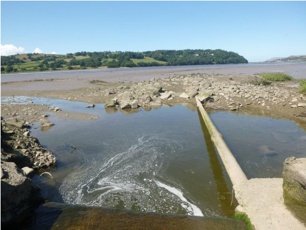
Photo 5 - Watercourse on upside (Taken 040822)
