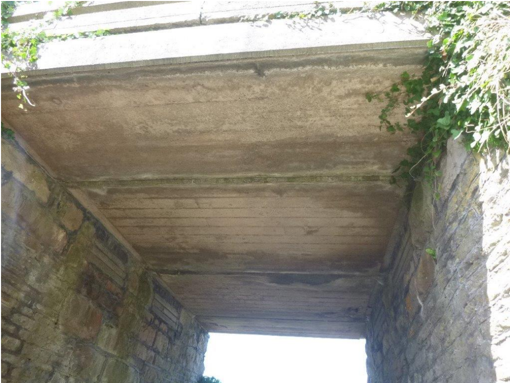
Photo 3 - Soffit general view (Taken 040822)
