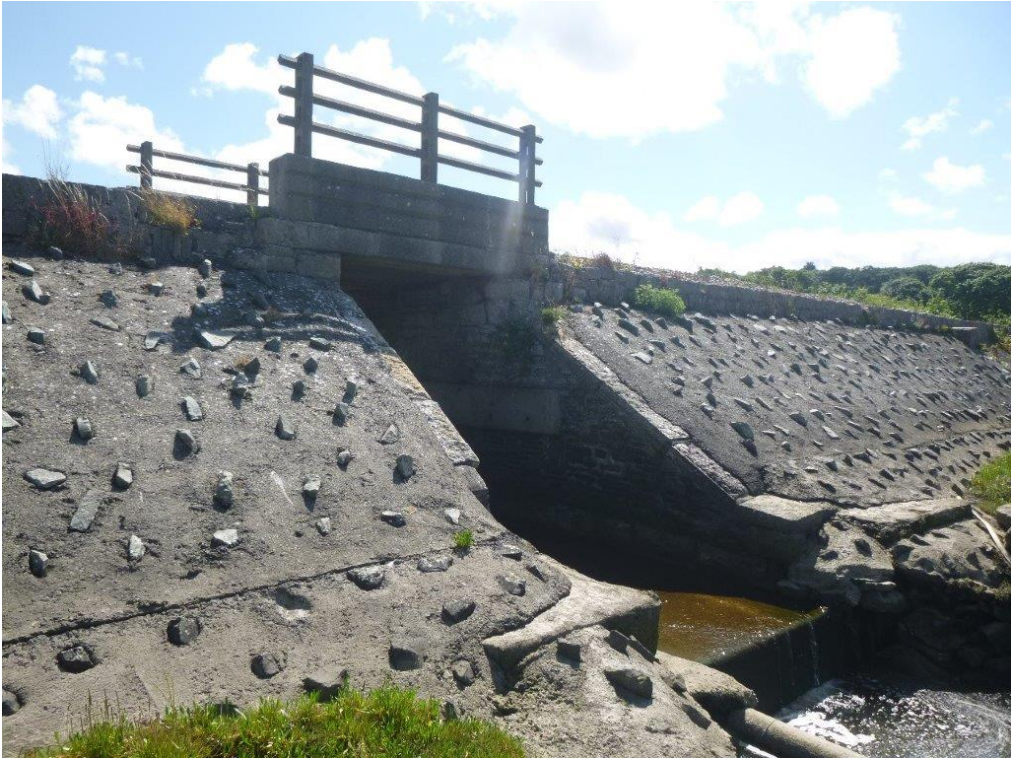
Photo 2 - Upside elevation (Taken 040822)
