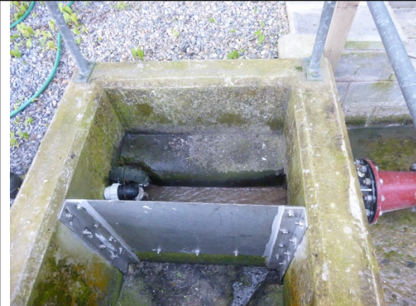
The inlet was free of debris and fungus.
