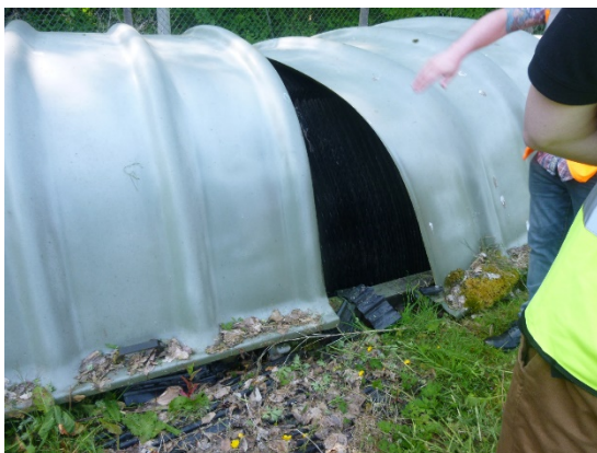
RBC in operation.
