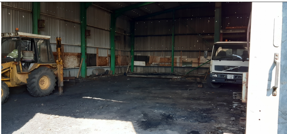
Photo 2 - Inside transfer station building / permitted area
