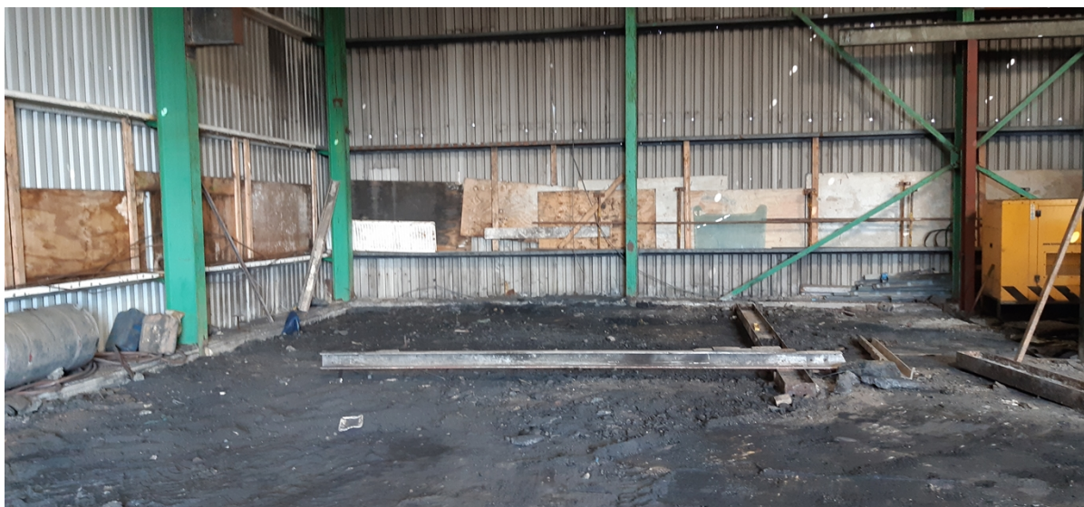
Photo 1 - Area where DCWW pipework runs through
