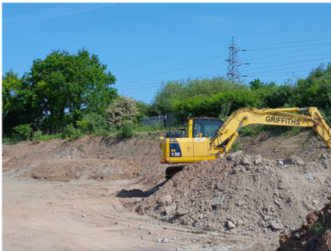
Photo 1 – Showing aggregate pile and excavator
