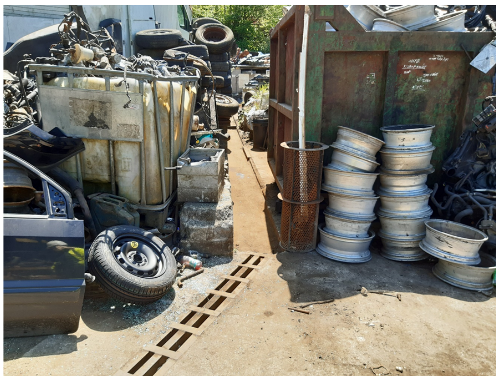
Photo 4 – drainage channels of area of engineered containment
