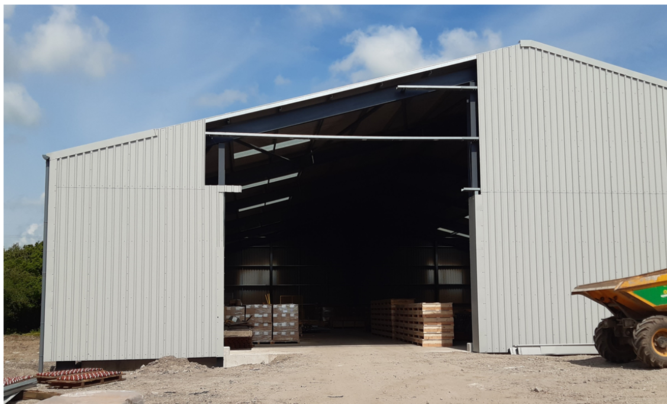
Covered swarf storage area under construction
